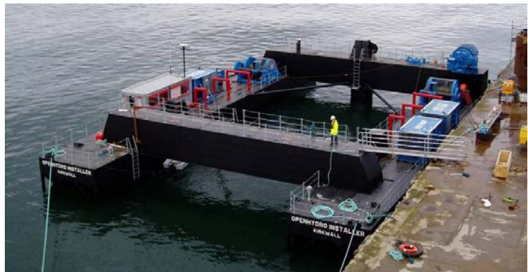
The OpenHydro Installer During Construction
