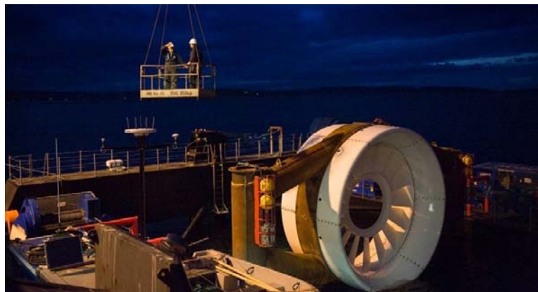
Open-Centre Turbine Being Prepared For Deployment In Orkney
