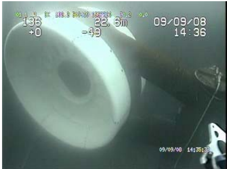
Completed Installation; Seabed Mounted Tidal Turbine
